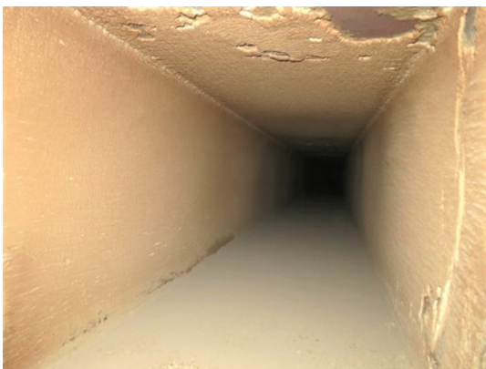
Furnace ash with resistant layer of tar
